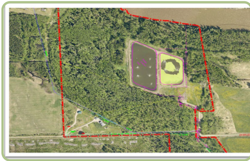
Aerial view of the Wastewater Treatment Plant
